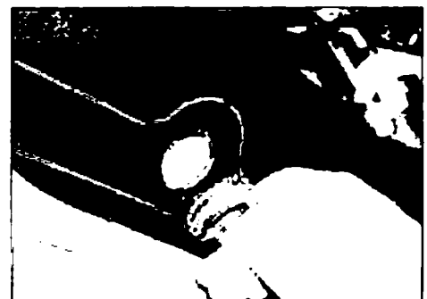
16.5b Check the sealing grommet condition
