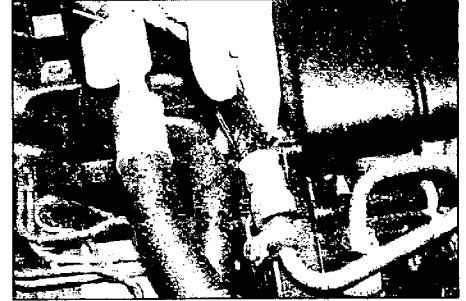
7.11 Check the condition of the power steering pump fluid hoses, paying particular attention to crimped unions
